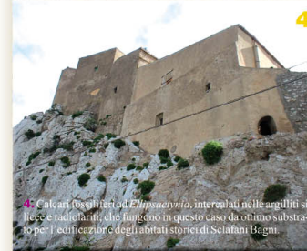
4. Ellipsacynia fossiliferous limestones, interbedded with siliceous argillites and radiolarites acting in this case, as foundation for the building of historical residential areas of Sclafani Bagni.
